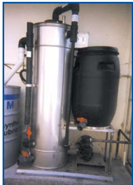
Oily Water Separator
